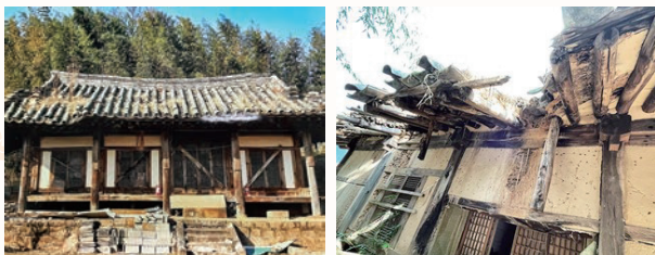
▲ The rafters of Yeongmojae are about to collapse because of the decay.
