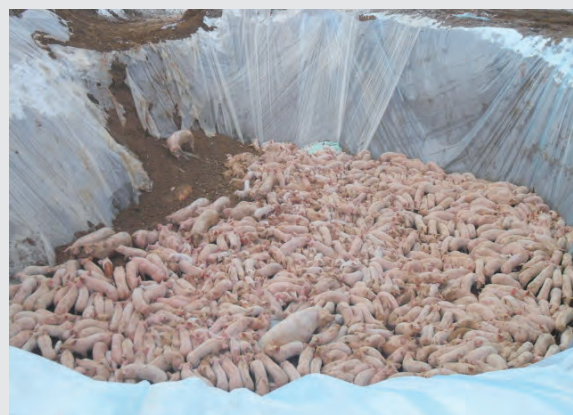
▲ To prevent leachate leakage, two layers of vinyl are placed at the bottom of the burial site before livestock is buried.
