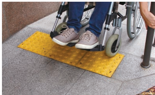
▲ Bumps in the end of the slope made for the blind can be an obstacle for the people in a wheelchair. It is not necessary for the blind because they usually use the stairs.
