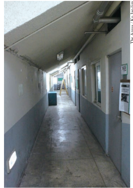
▲ The inside of the underground of the Open Air Theater
