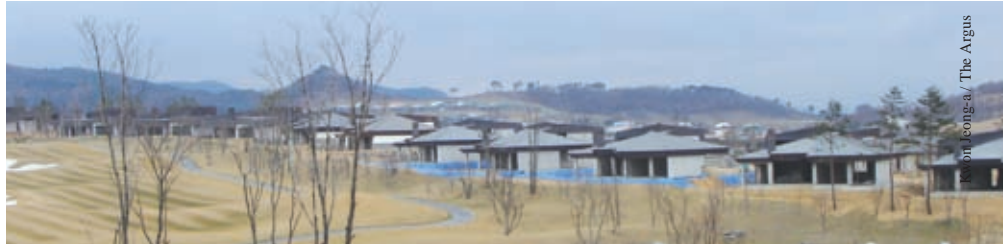
There was still construction going on, despite it being the weekend.
