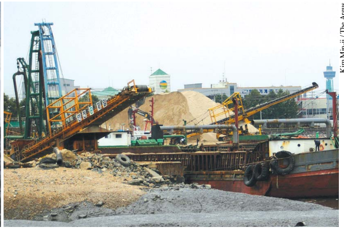
Ships are ready to move the sand to the sea to reclaim the tidal land.
