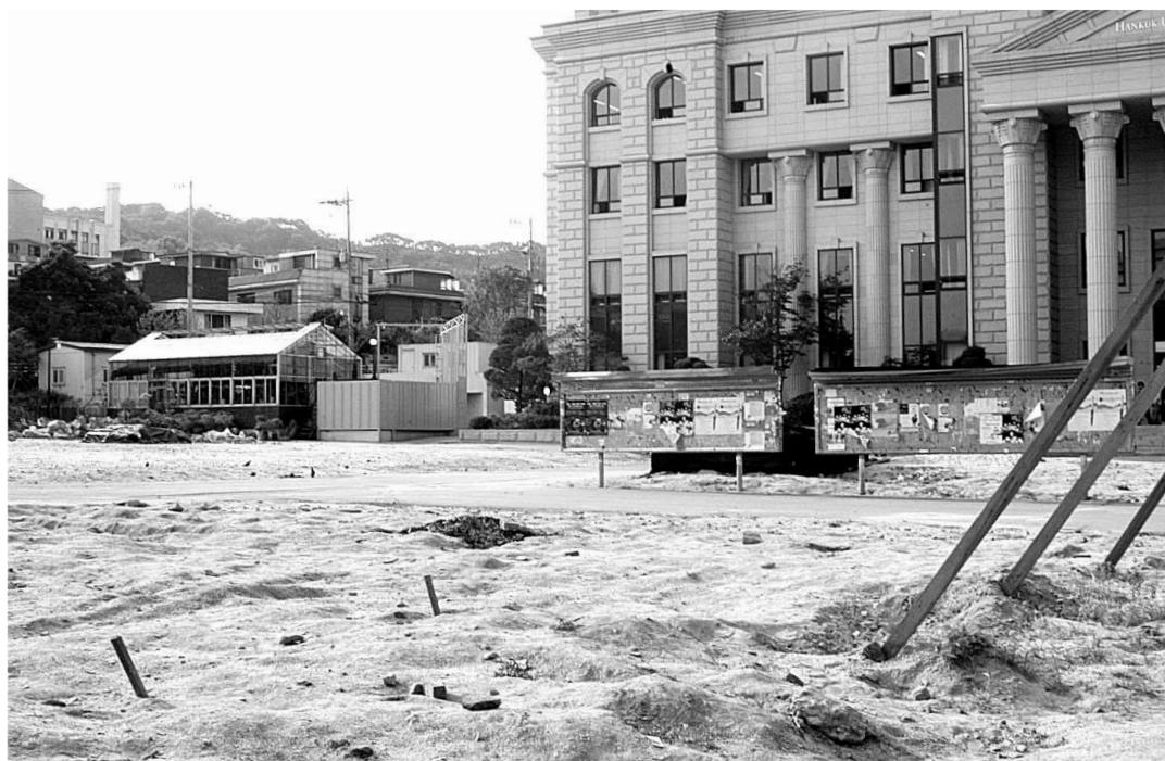
Dormitory construction will begin here in October.
