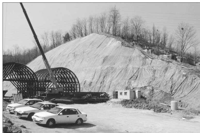
There are still many unauthorized houses near the main stadium.
